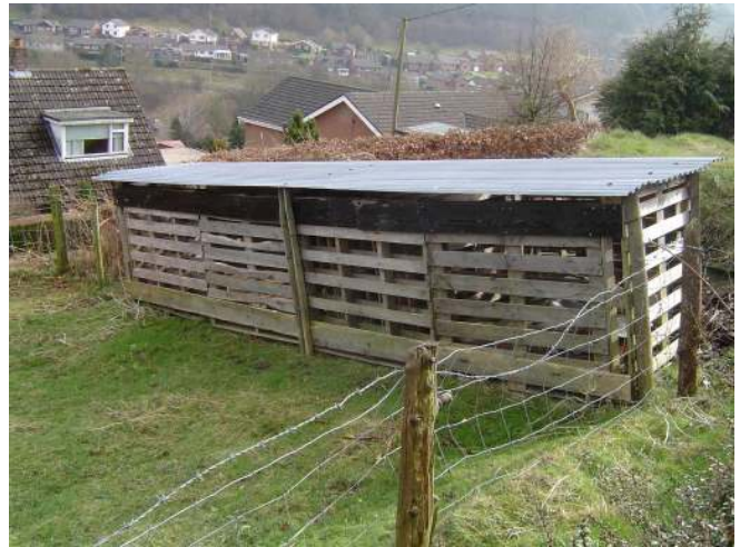
One KTAT Trustee's low-cost wood drying shed made from (mostly) recycled materials.
